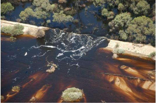
Figure 2: Levee failure in Lower Loddon
